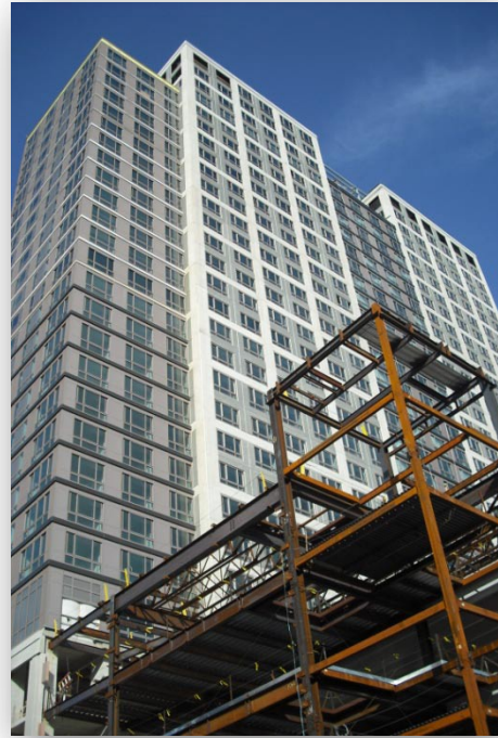
Figure 30: Under Construction – April 2010
