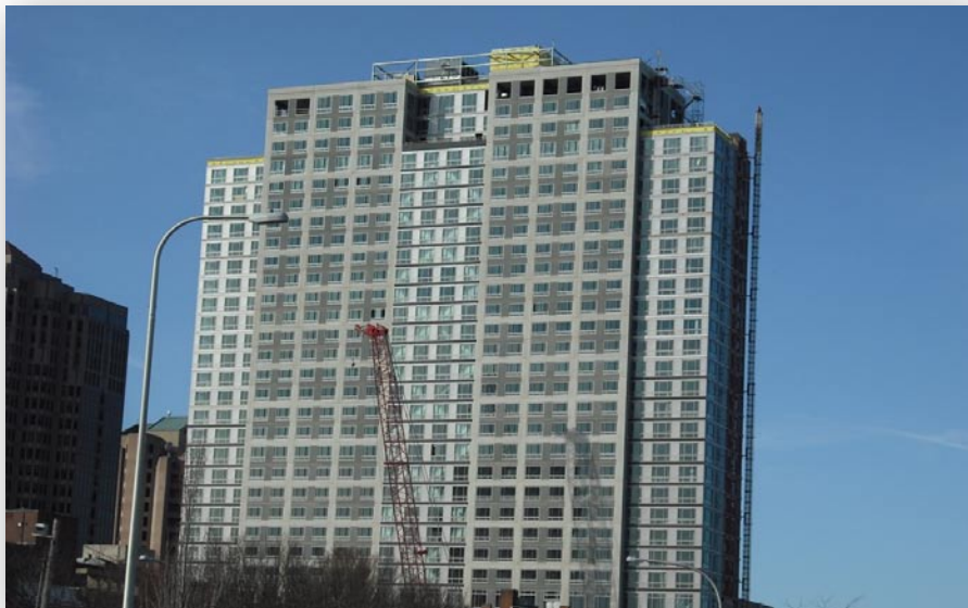
Figure 1: Most recent image of 360 State Street under construction- April 2010.
